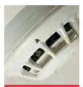
In addition to break glass points, protection must be provided by means of automatic heat/smoke detectors.
