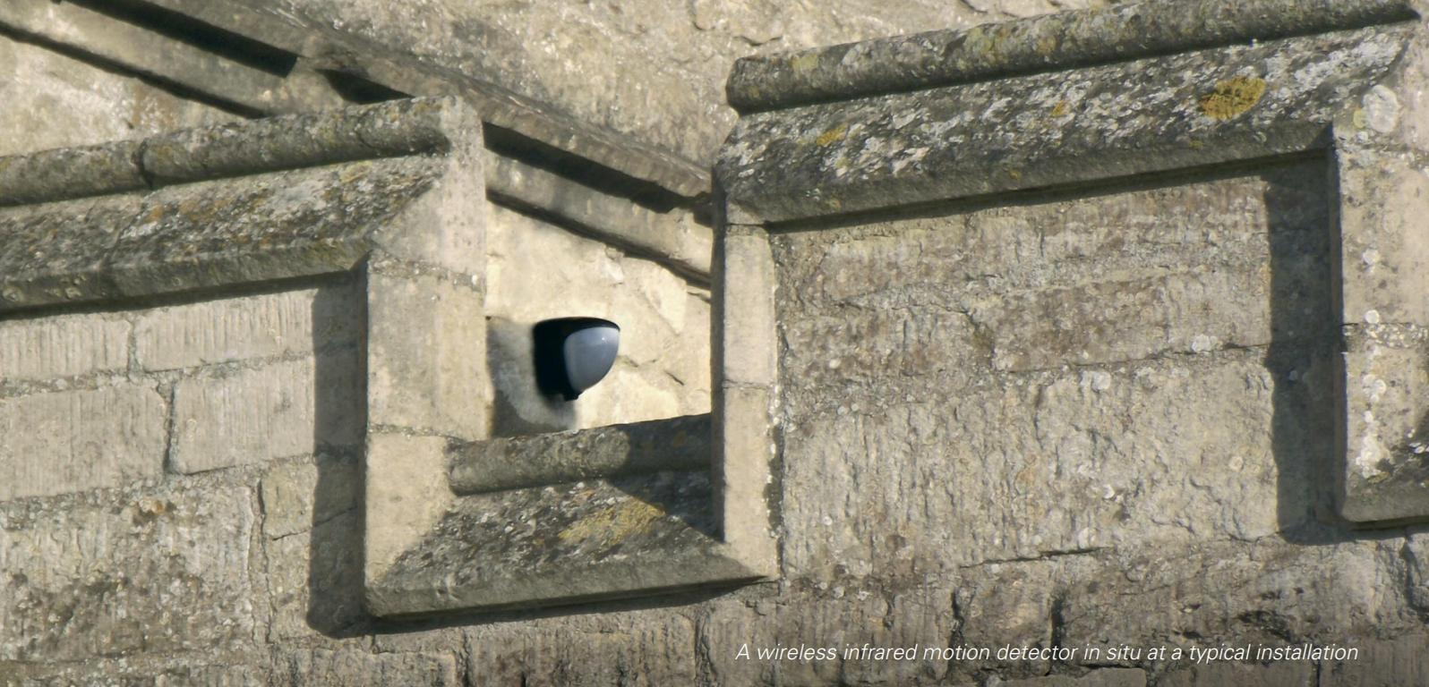
*A wireless infrared motion detector in situ at a typical installation*
