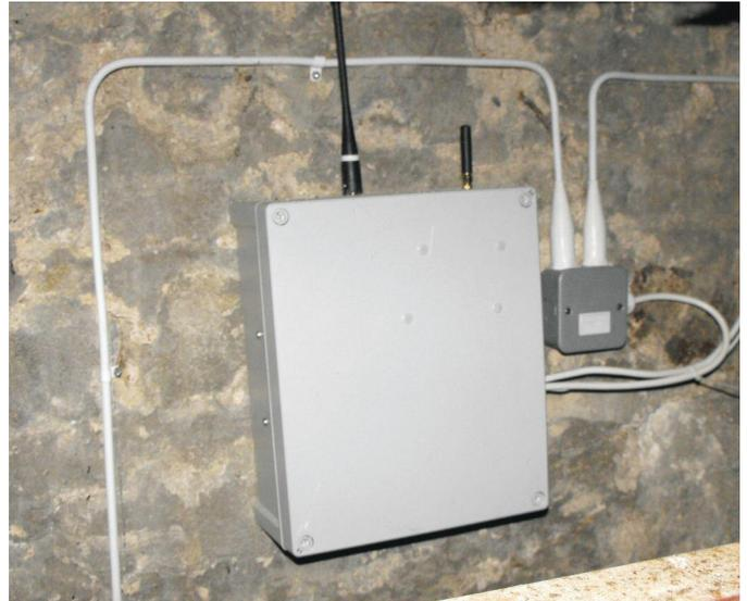
*Roof security system panel installed in a church tower*
