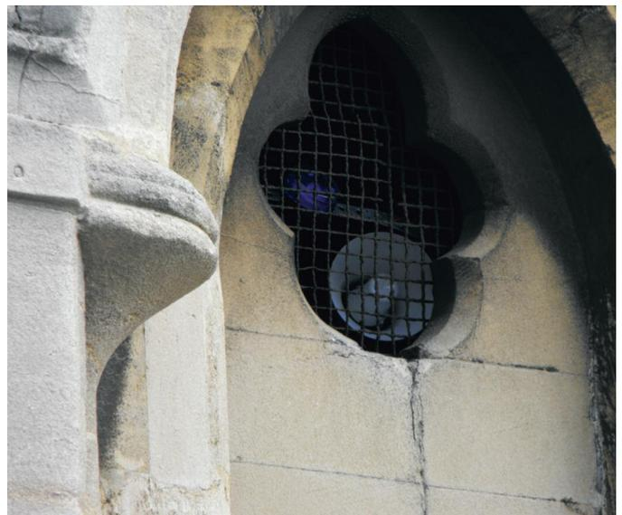
*Alarm sounder and blue strobe light installed in a church tower*
